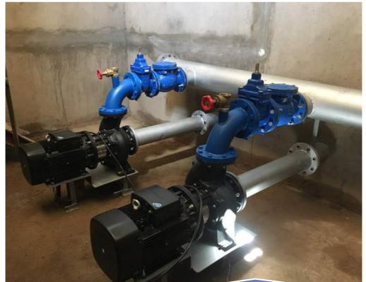
Use of Standard AC pumps up to 37kW, either submersible or surface.
